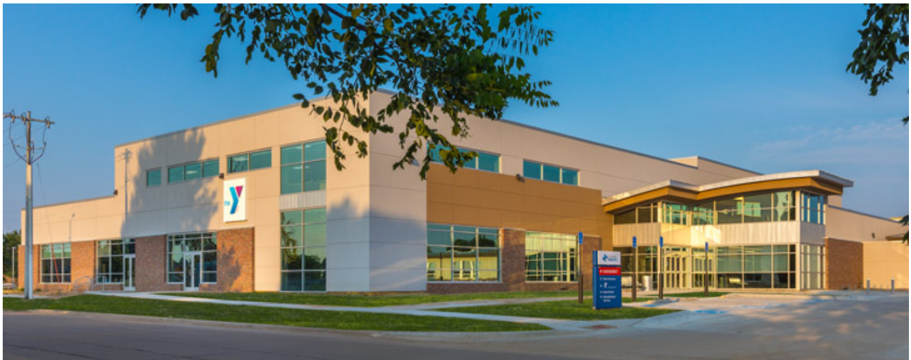
In the small town of Gothenburg, Nebraska, the hospital is co-located with a YMCA.
