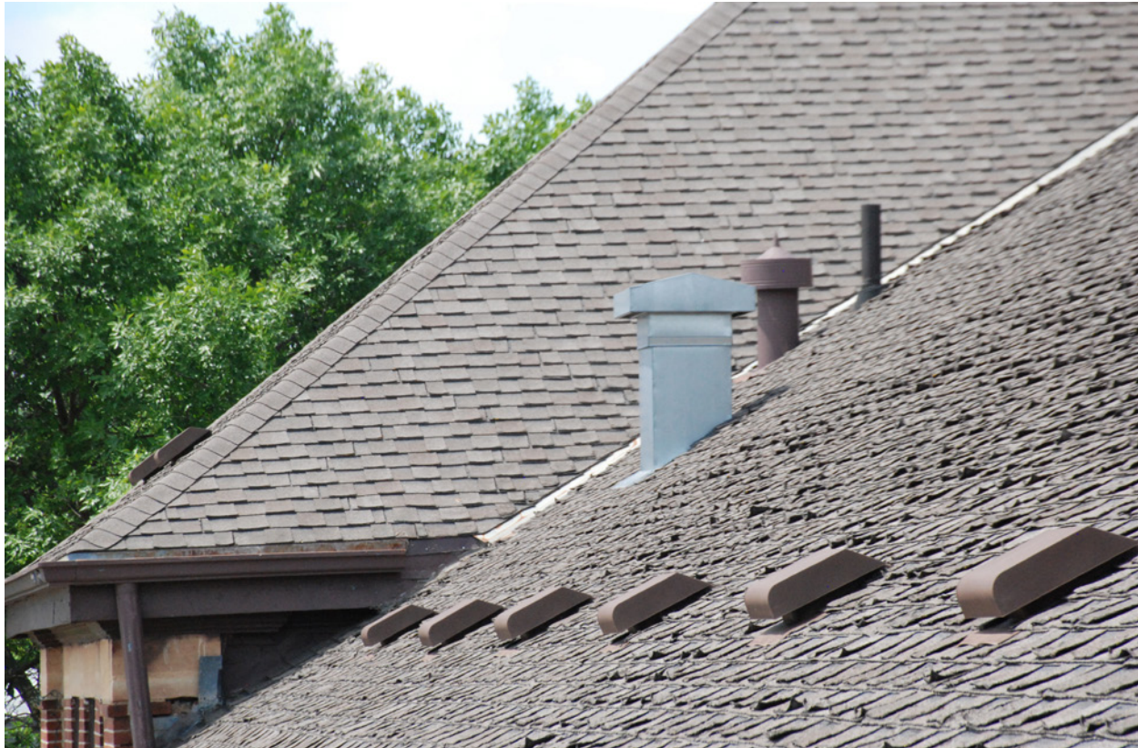
8 Shingle roof—condition of shingles at south elevation. June 2018.
