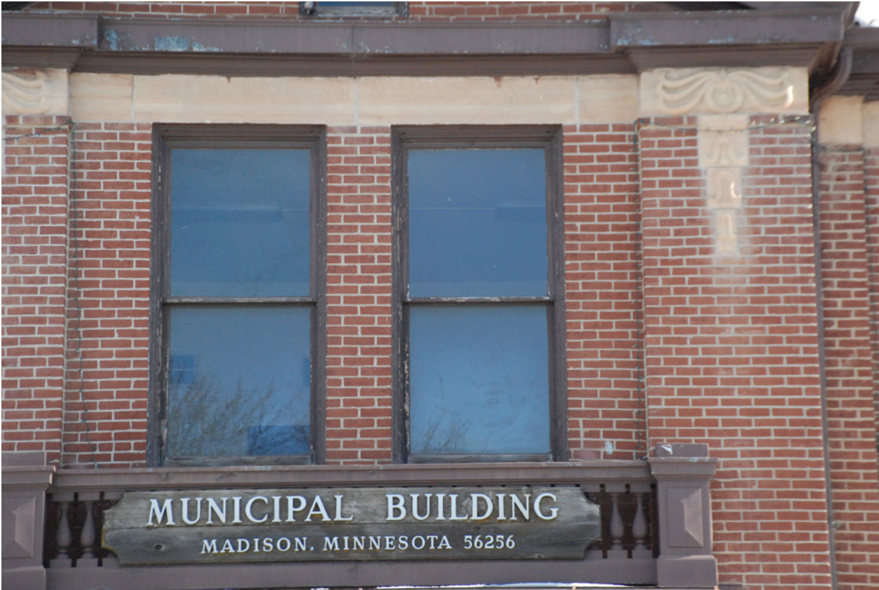
26 Typical pair of double-hung windows, west elevation. June 2018.
