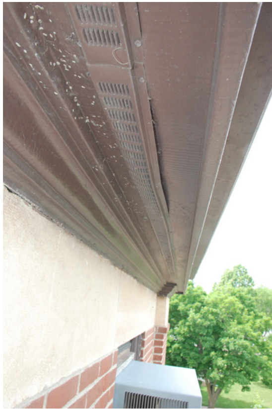
13 View of existing venting at underside of soffit. June 2018.
