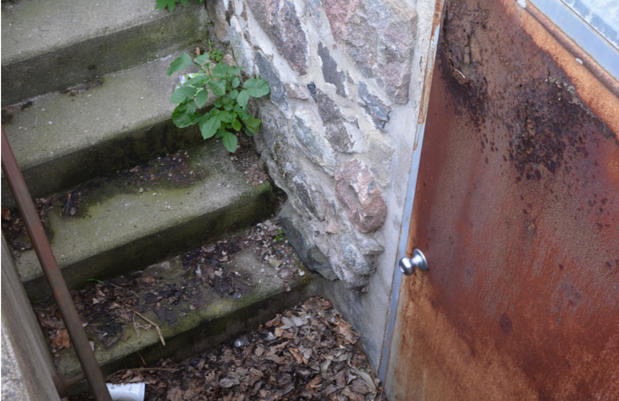
25 Concrete stair and door to basement at north elevation. June 2018.
