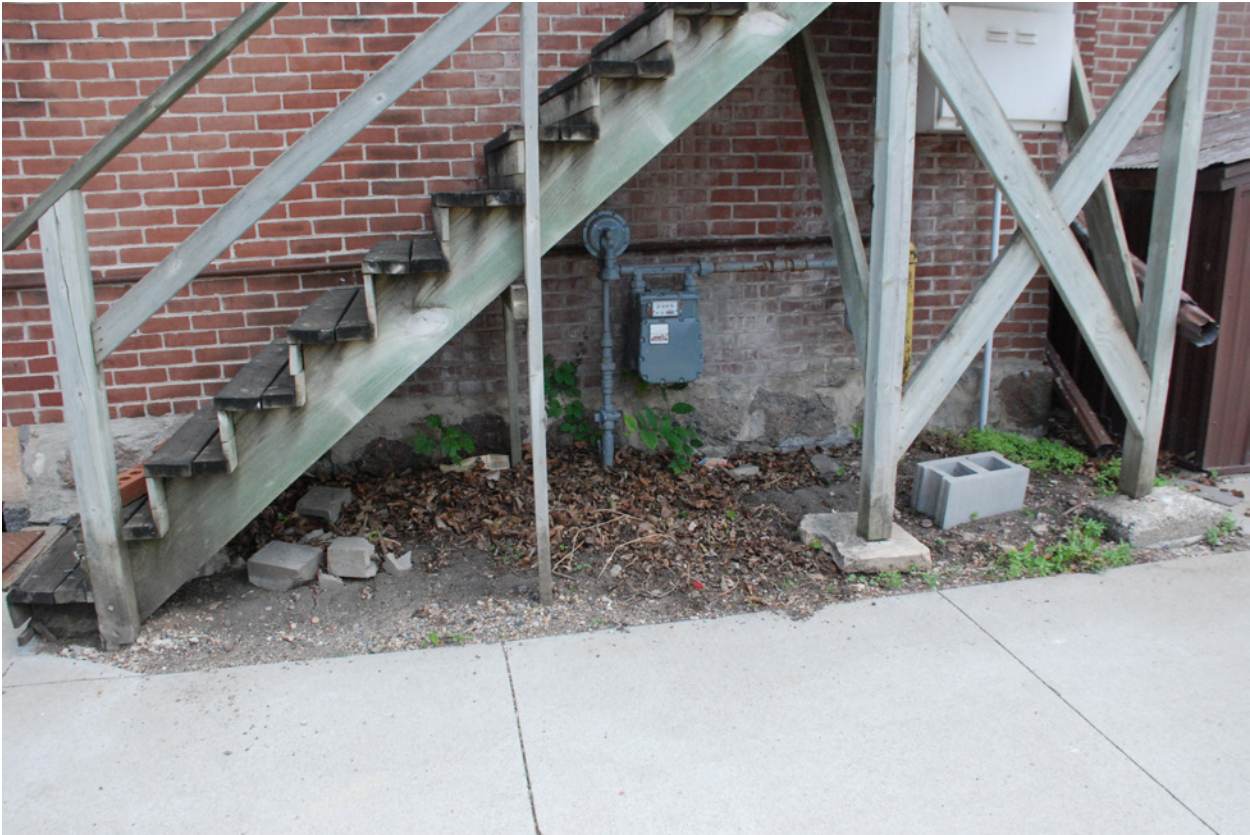
36 Existing stair at north elevation to be removed. June 2018.
