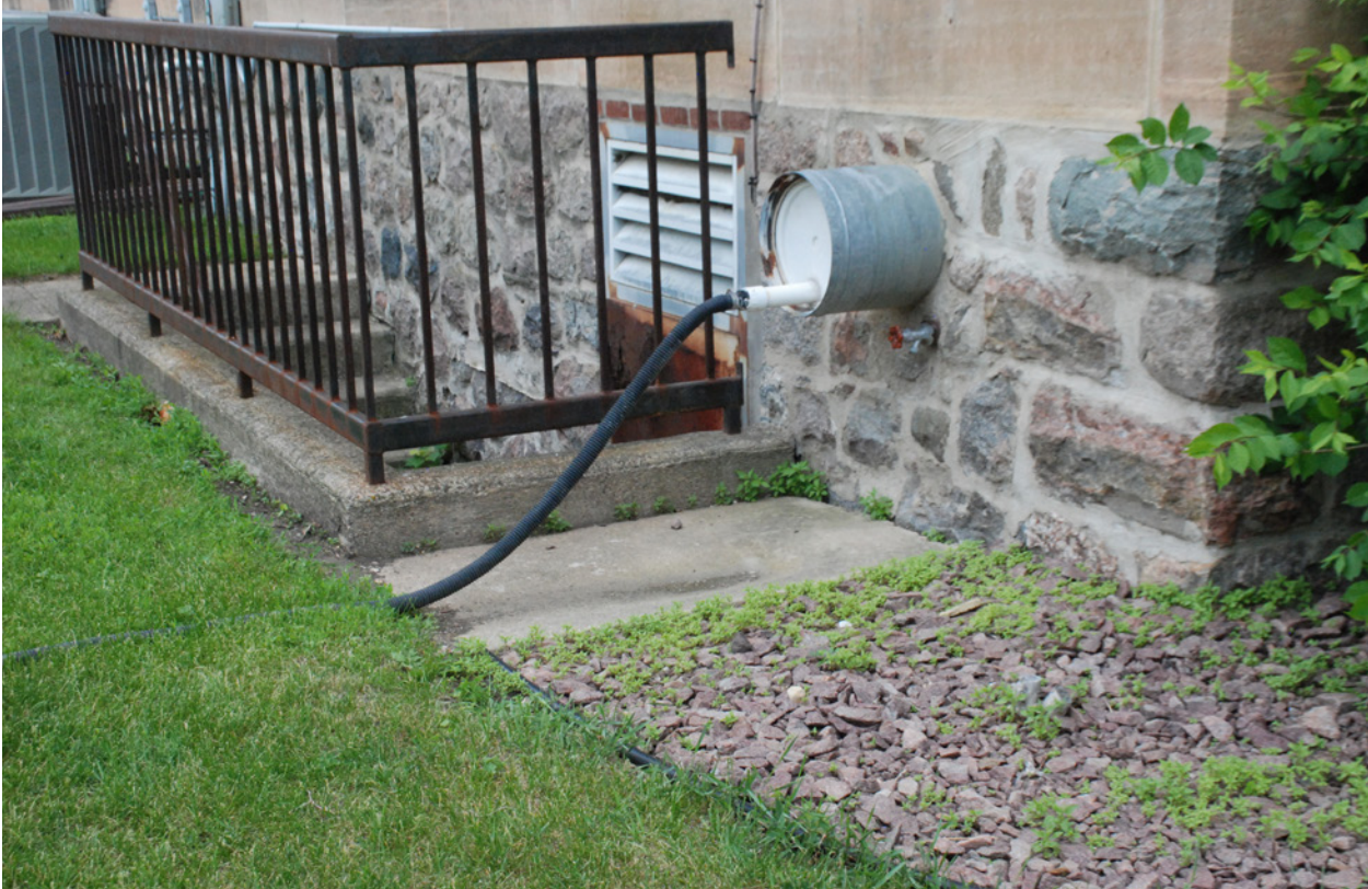
33 Northwest corner of building; guard rail and sump pump drain. June 2018.
