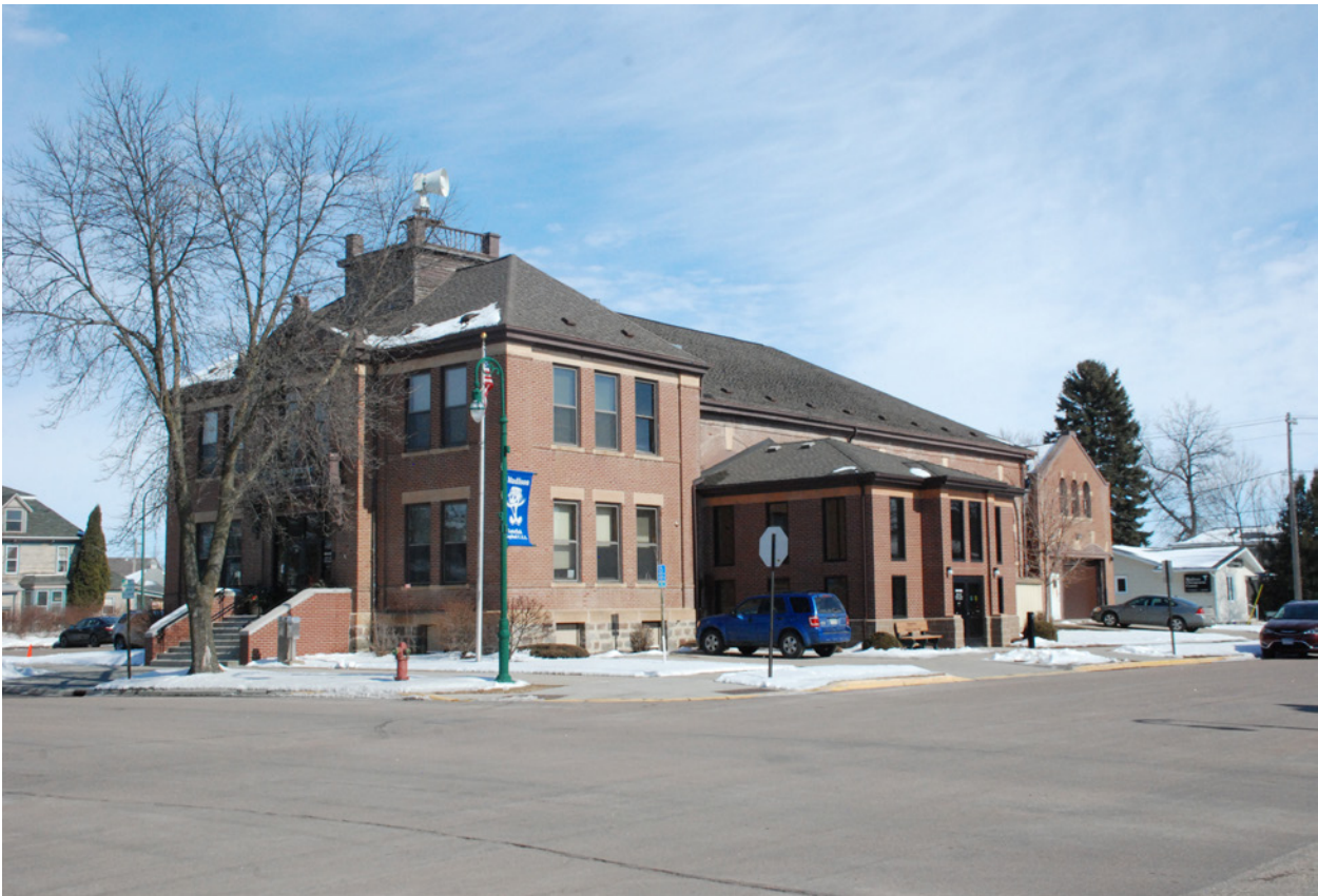
3 City Hall, south elevation.
