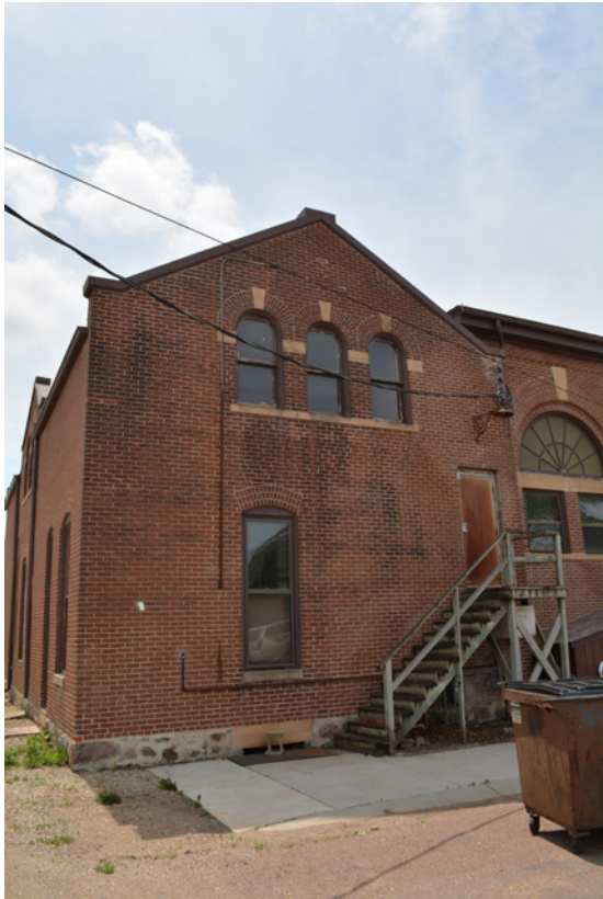
6 Firehouse, north elevation. June 2018.
