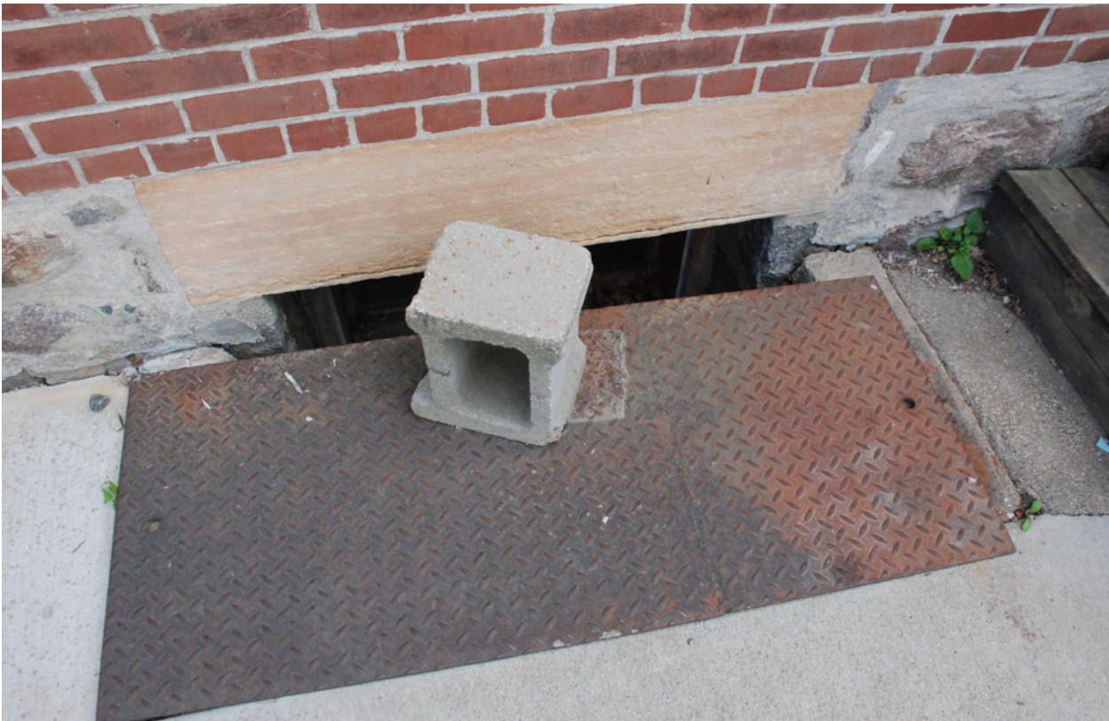
35 Metal plate covering window well at Firehouse, north elevation. June 2018.
