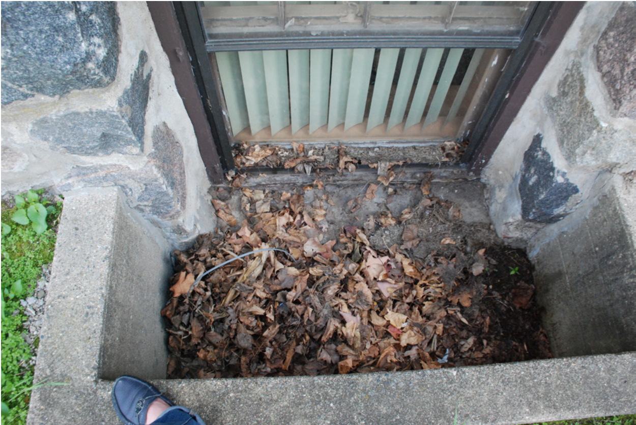
32 Typical basement window and well. June 2018.
