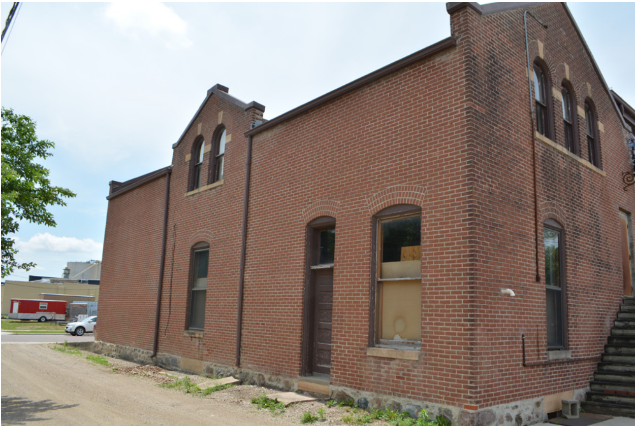
5 Firehouse, east elevation. June 2018.
