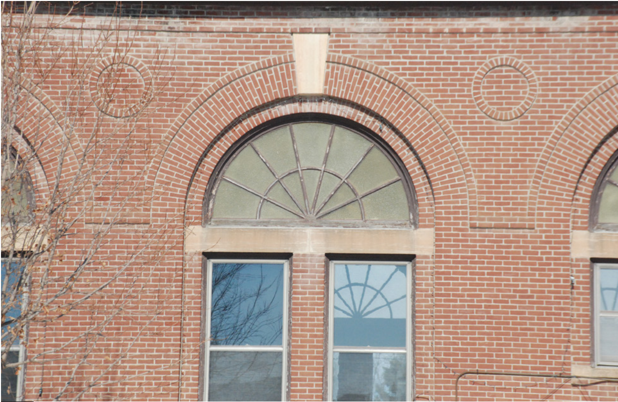
27 Typical arch window over pair of double-hung windows, south elevation. June 2018.
