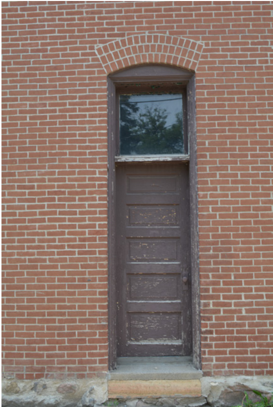
24 Existing door at Firehouse, east elevation. June 2018.
