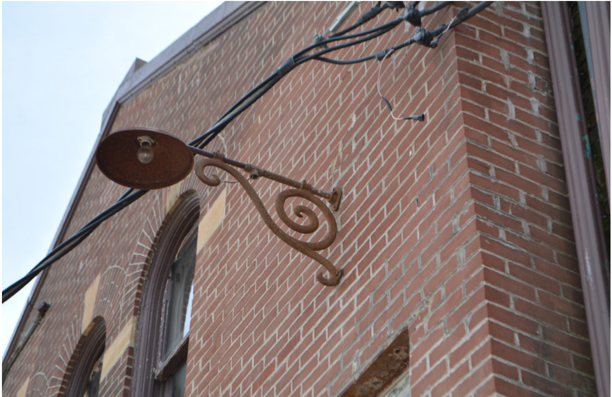
37 Existing light fixture at north elevation, to be repainted. June 2018.
