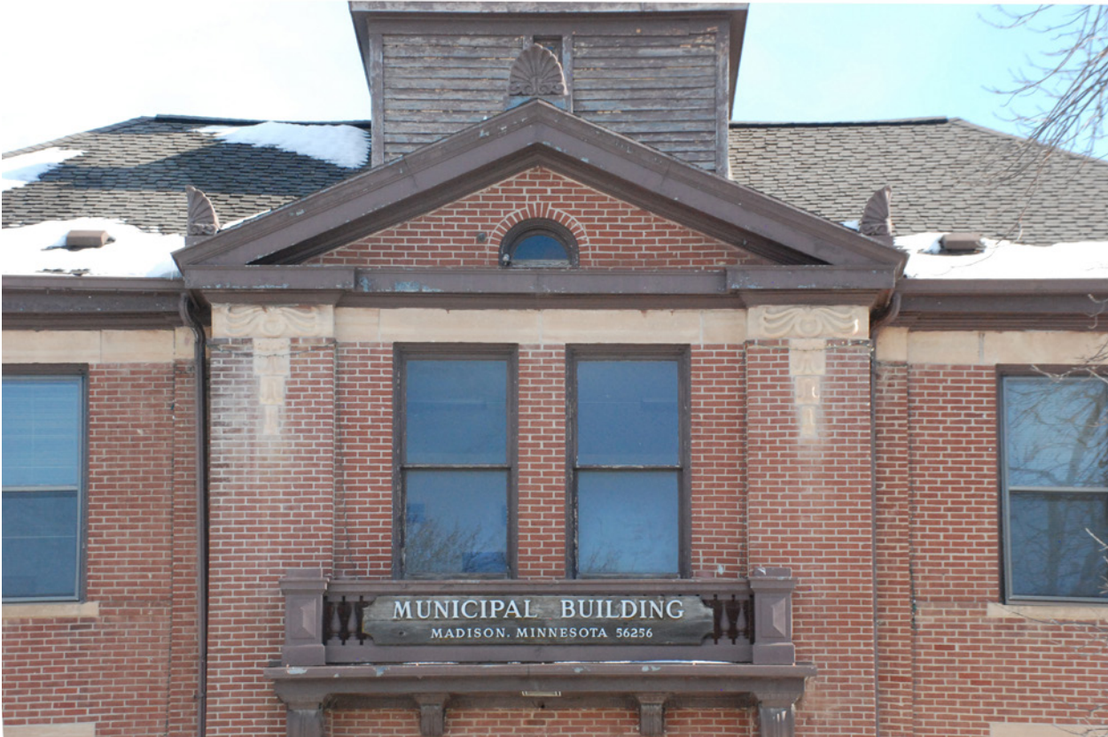
18 View of balcony over main entry at west elevation. June 2018.
