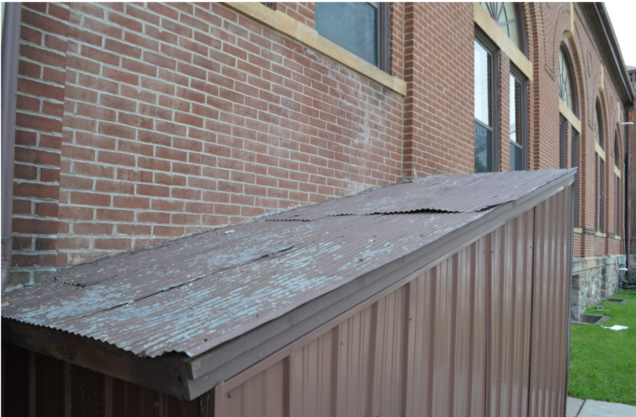
17 Top of corrugated metal roof, north elevation. June 2018.
