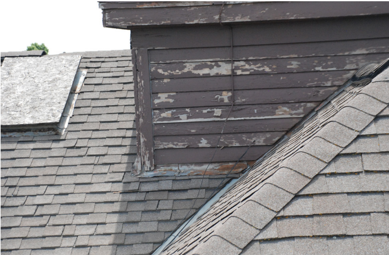
9 Existing roof hatch, north elevation. June 2018.
