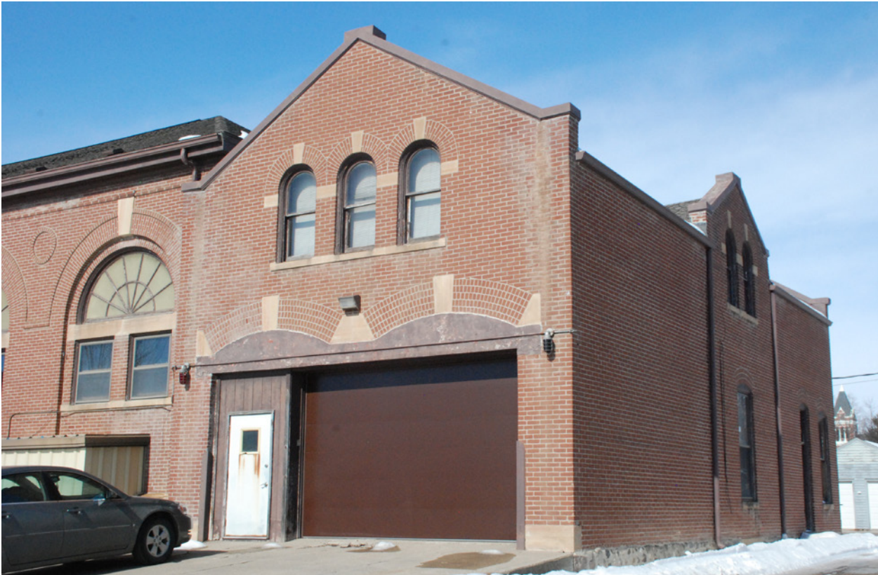
4 Firehouse, south elevation.
